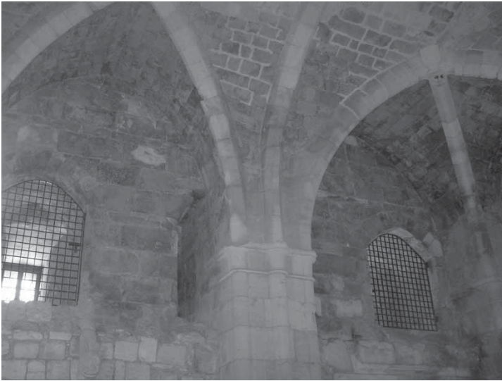
Fig. 41: Limassol Castle, réduit , upper part of western wall and rib-vaulting [M. Olympios].
